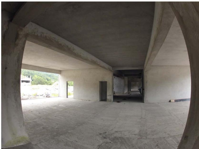
PISO TÉRREO DO BLOCO "A" ALVENARIA E REBOCO PARCIALMENTE CONCLUÍDOS
